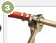
3 Tighten compression union onto aluminum line
